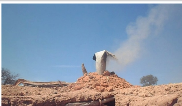
Plate 7: Smoke and dust from ICS are fully controlled and directed outside the kitchen environment through the chimney.
