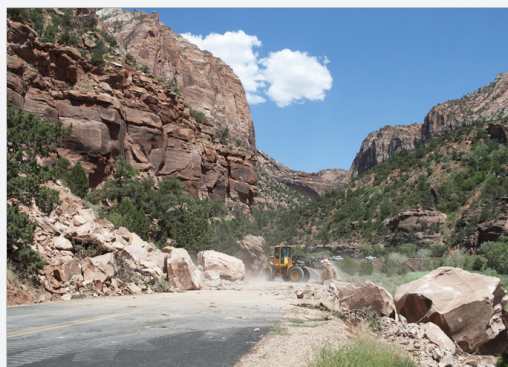
Figure 1: Rockfall on a road from the adjacent slope.
