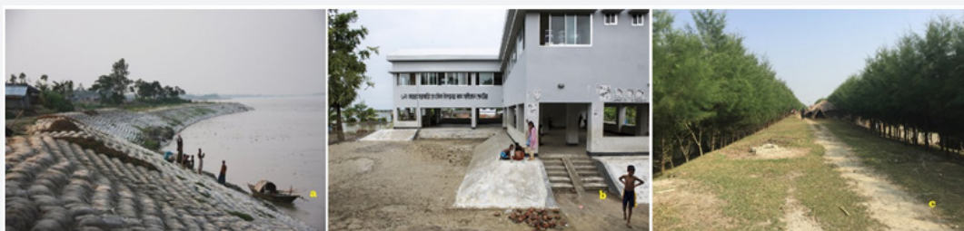
Figure 6: Different types of structural adaptation to sea level rise in the coastline of Bangladesh:
