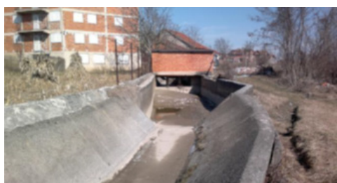
Figure 4: Current state of Zdunje-Pirok channel- urban area. (Source: [24]).
