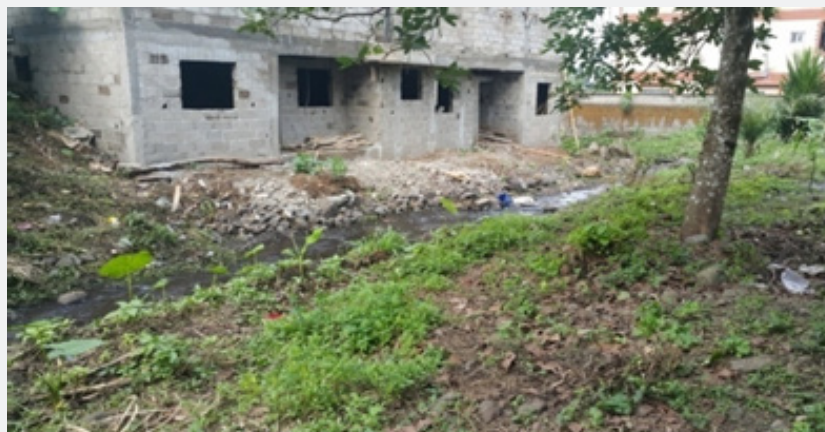
Figure 5: Construction site Koke (4°10'22.639" N, 9°16'45.693" E).
