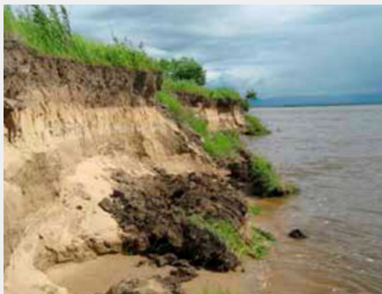
Figure 8: Erosion and associated landslide-rockfall phenomena on the banks of the lower reaches of the Amur River.
