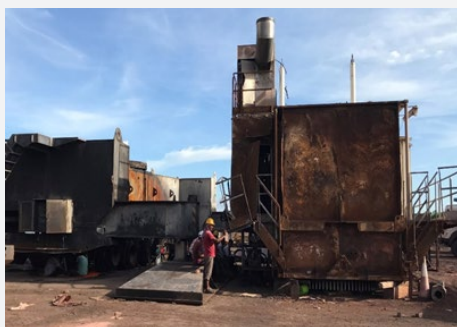
Figure 2: The front view of the burnt crane.
